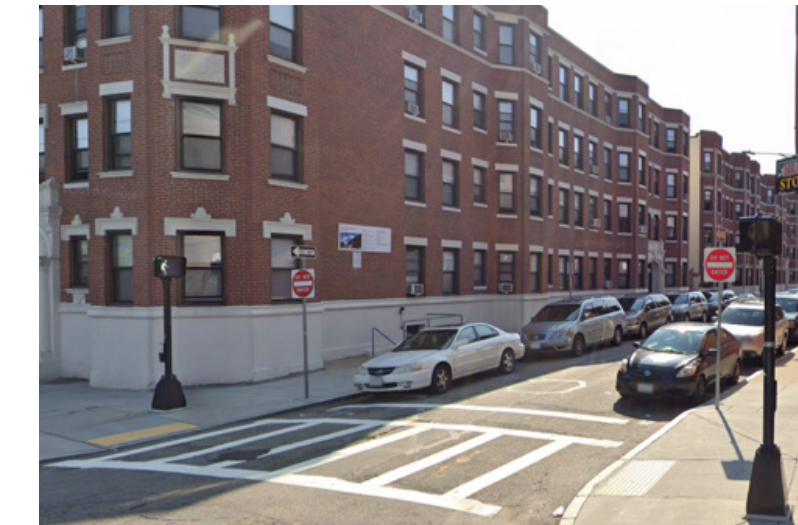
New crosswalk Blue Hill Ave. and Castlegate
