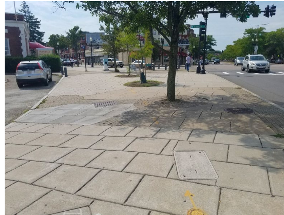
The renovated Unity plaza
