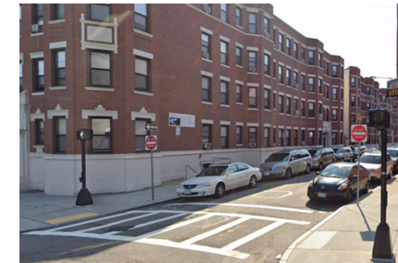
New crosswalk Blue Hill Ave. and Castlegate
