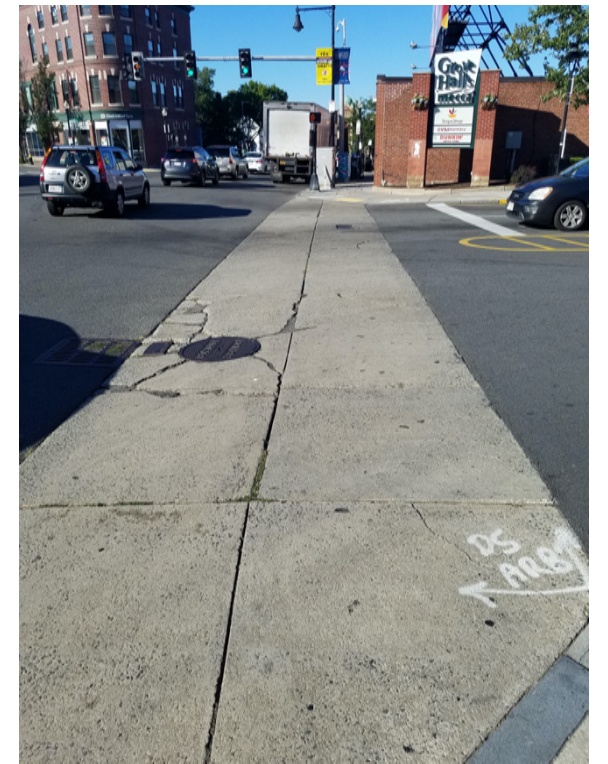
Crosswalk needed to cross Georgia St. on Blue Hill Ave. on the Grove Hall Mecca side
