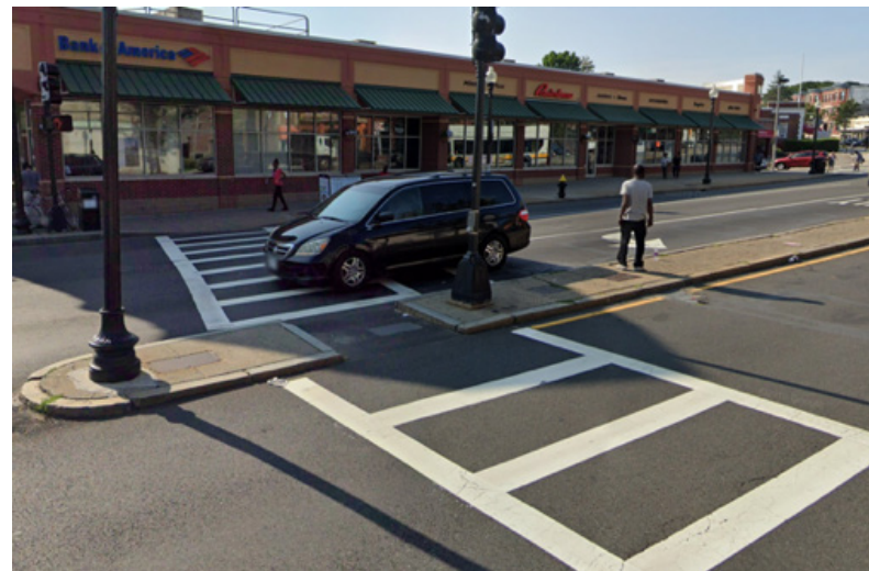
After pothole filling and resurfacing
