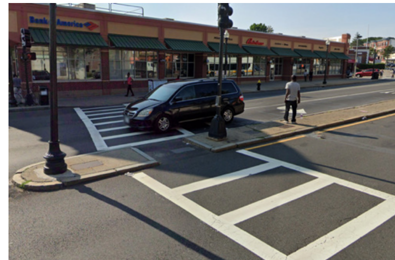
After pothole filling and resurfacing
