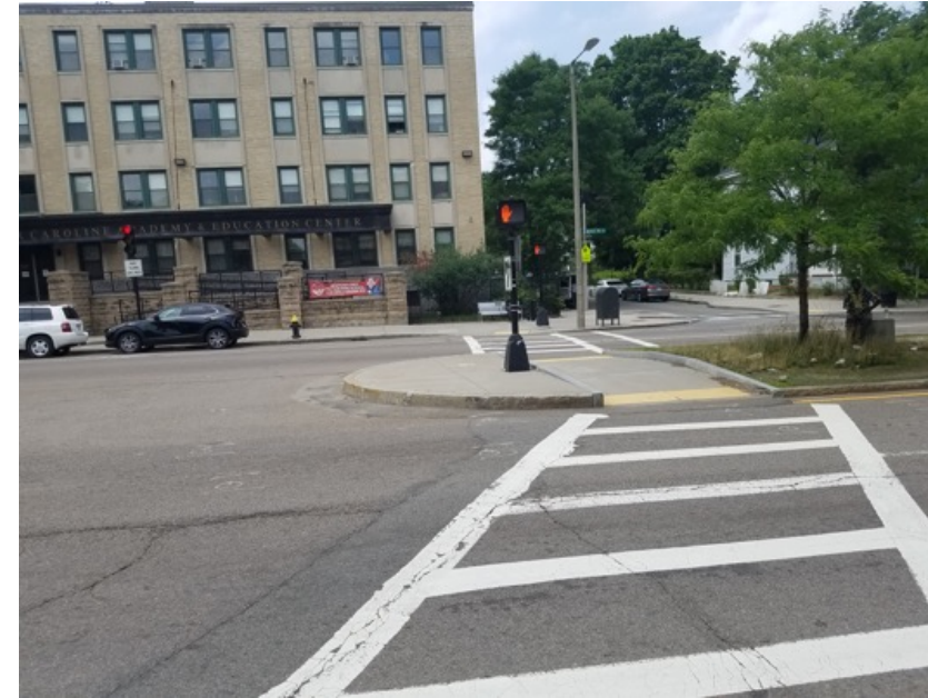
New crosswalk and traffic calming near Mother Caroline Academy
