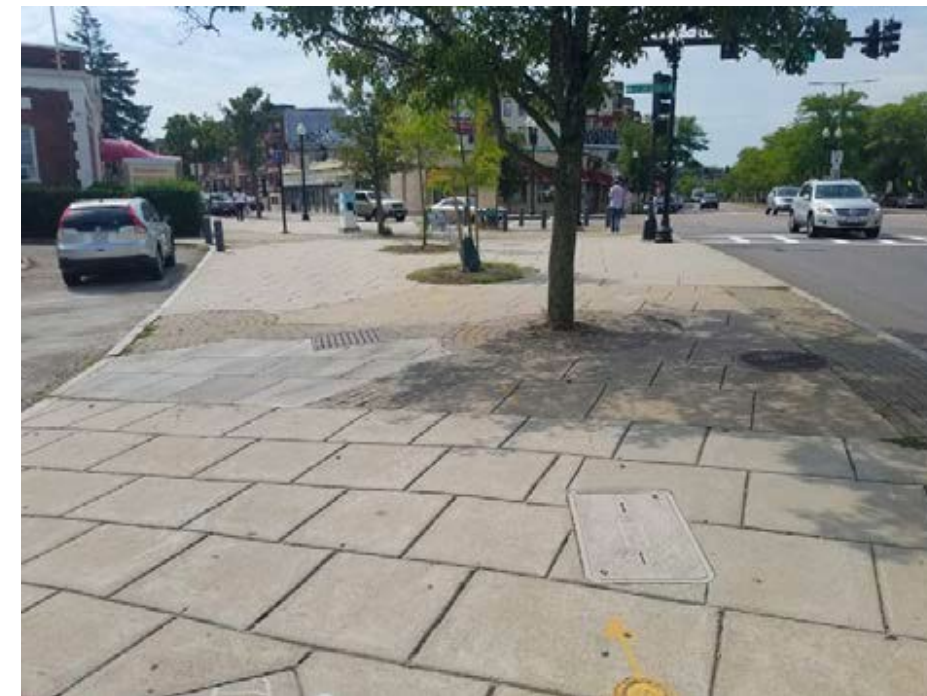
The renovated Unity plaza
