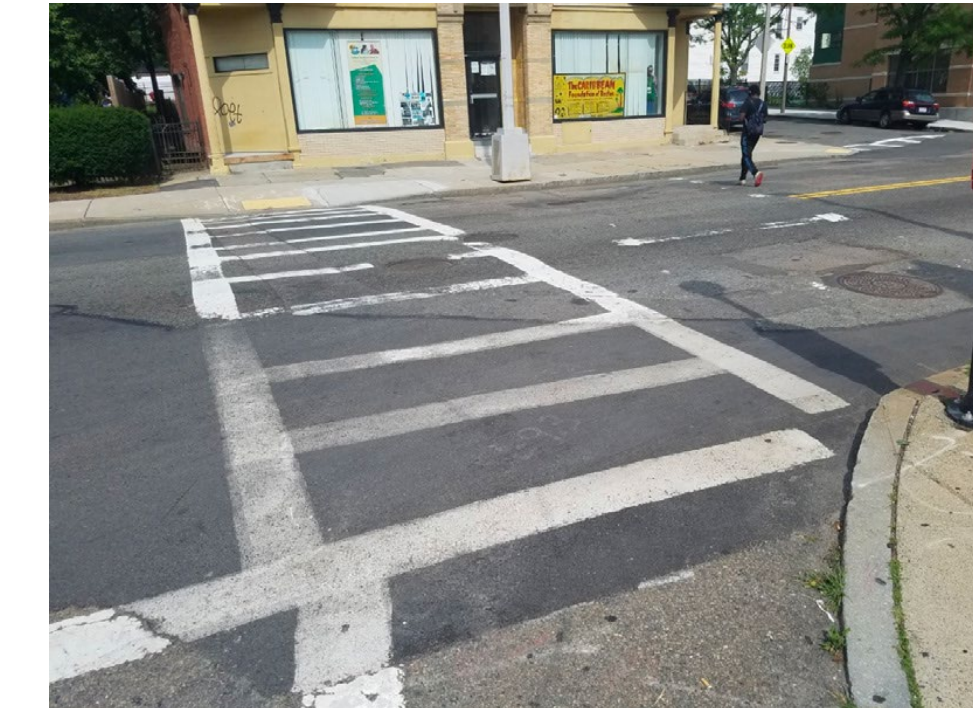
New crosswalk striping leading to the ADA accessible curb cut
