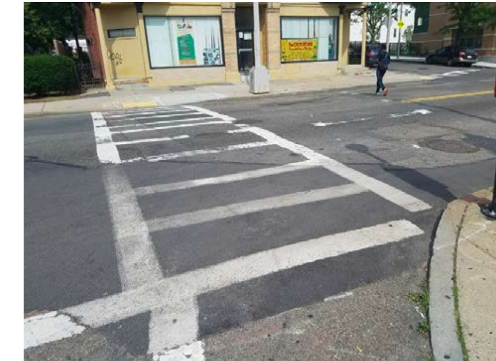
New crosswalk stripping leading to the ADA accessible curb cut
