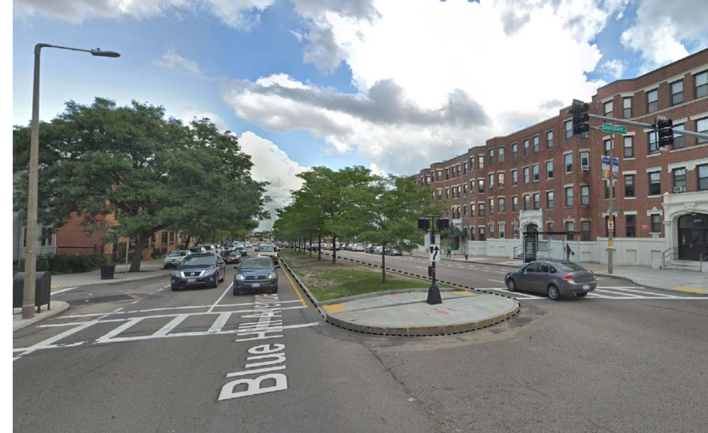
South end of the project median with a pedestrian crosswalk and adjacent bus stop.
