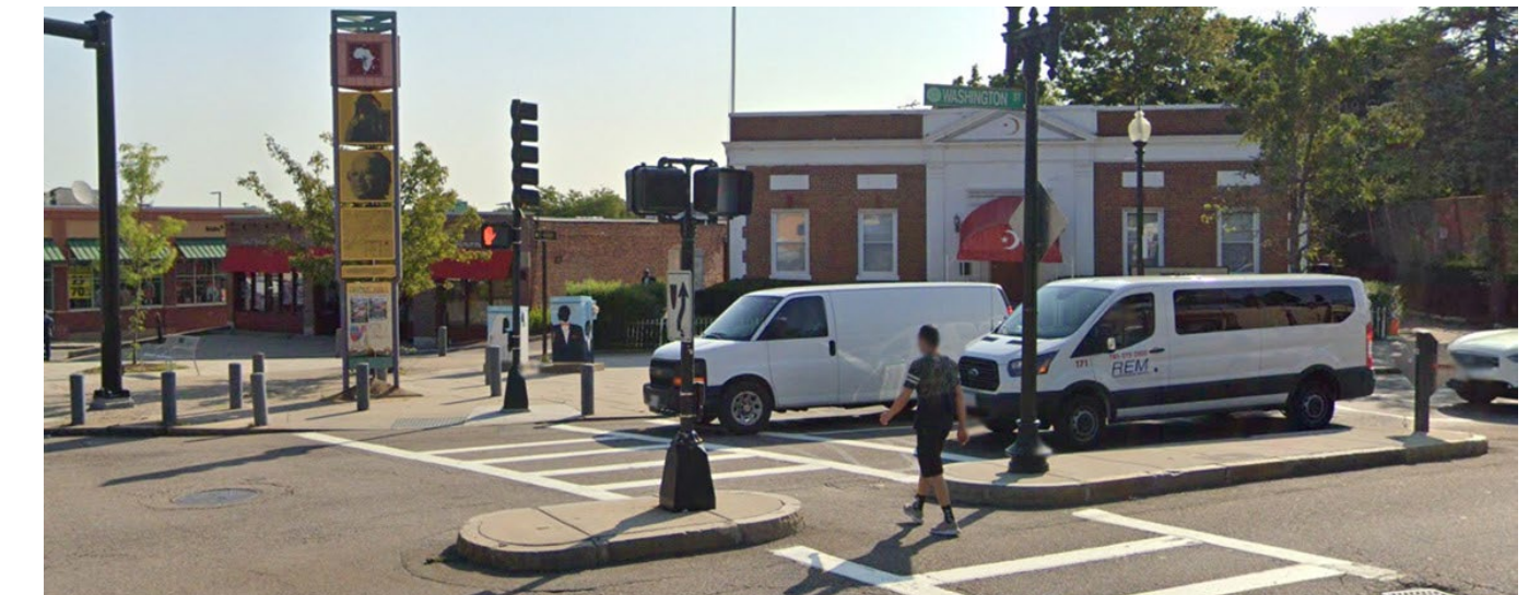
Pylon and island fixed
