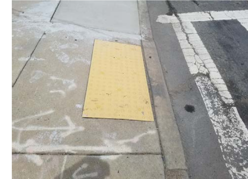
Example of Handicap Compliant Sidewalks
