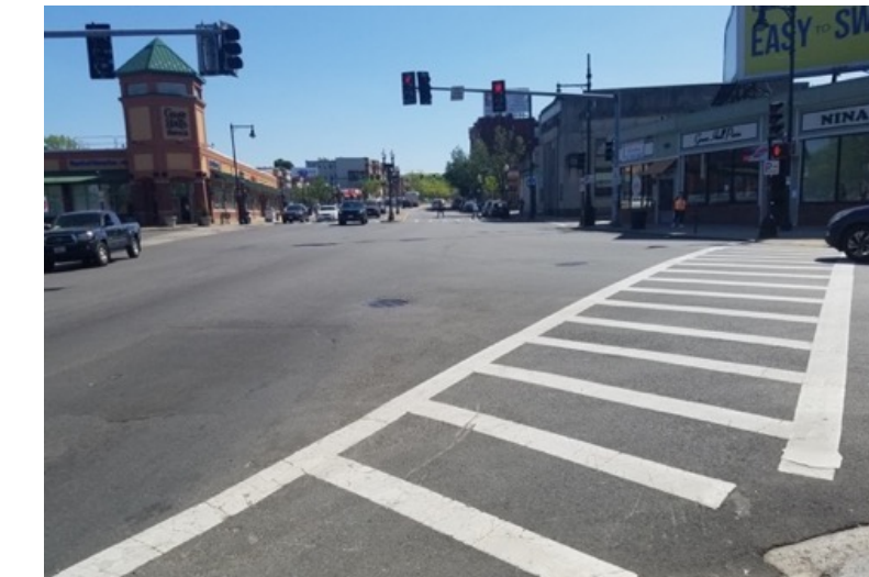
Resurfaced intersection at Blue Hill Ave. and Warren St.
