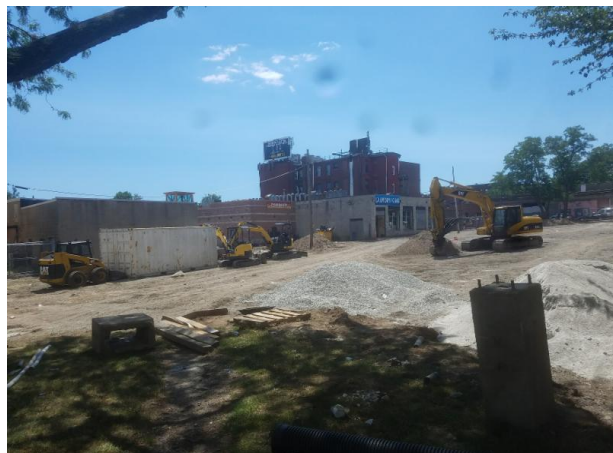
Another photo of pocket park and parking lot construction.
